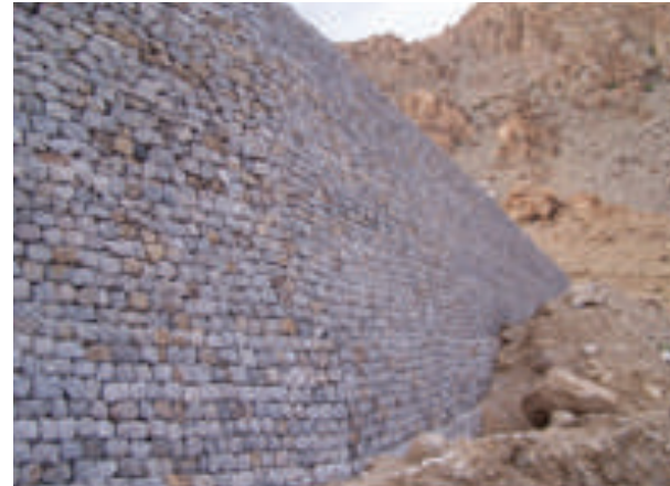
Figure 2: Retaining wall of the reservoir
